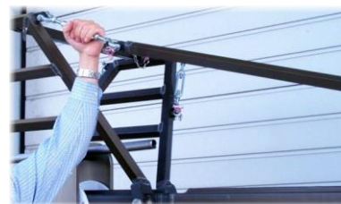
Tensioning the turnbuckle
